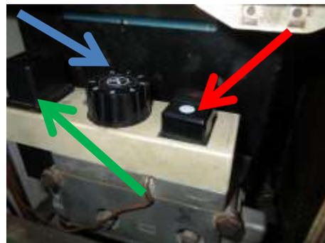
To turn on radiator circulation pump put the switch in the airing cupboard in the down position
